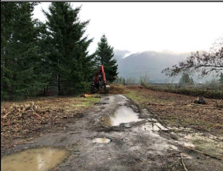
Excavation of test-pit TP-12, looking southwest
