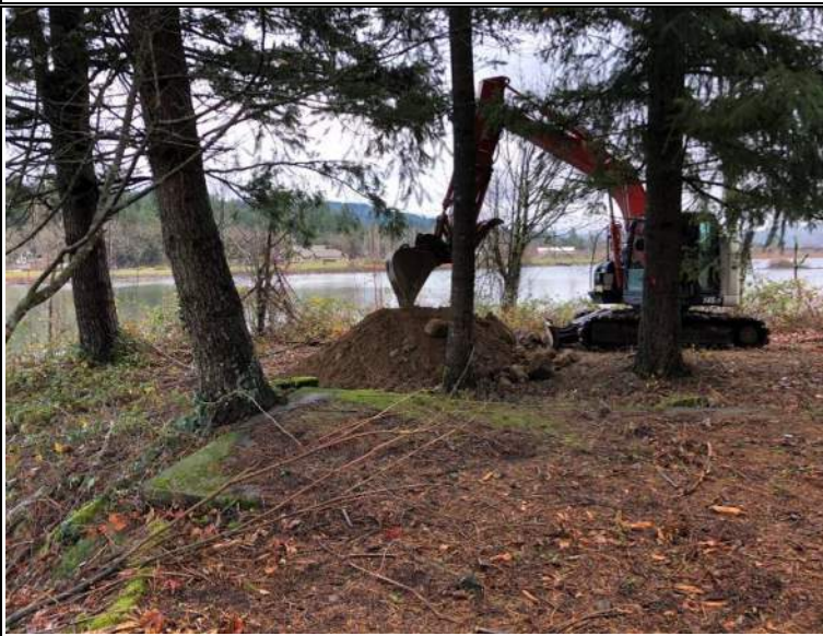
Excavation of test-pit TP-5, looking east
