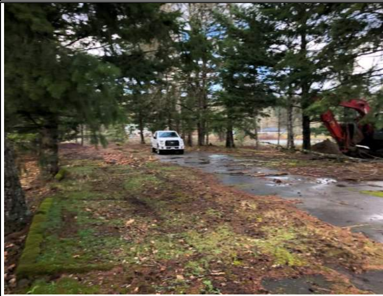
Excavation of test-pit TP-6, looking north
