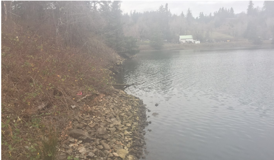
Photo 3. Riprap on the eastern shoreline, facing north.
