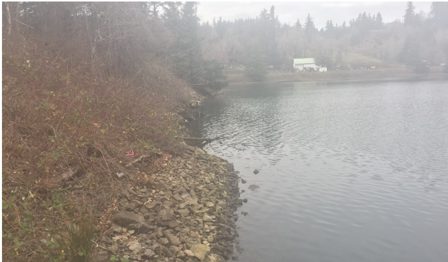
Photo 3. Riprap on the eastern shoreline, facing north.
