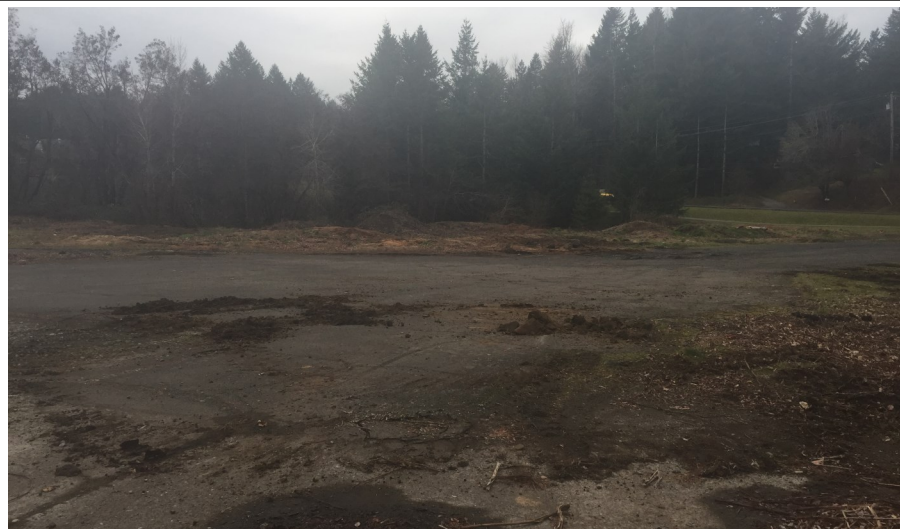
Photo 2. Existing concrete and gravel surfacing.
