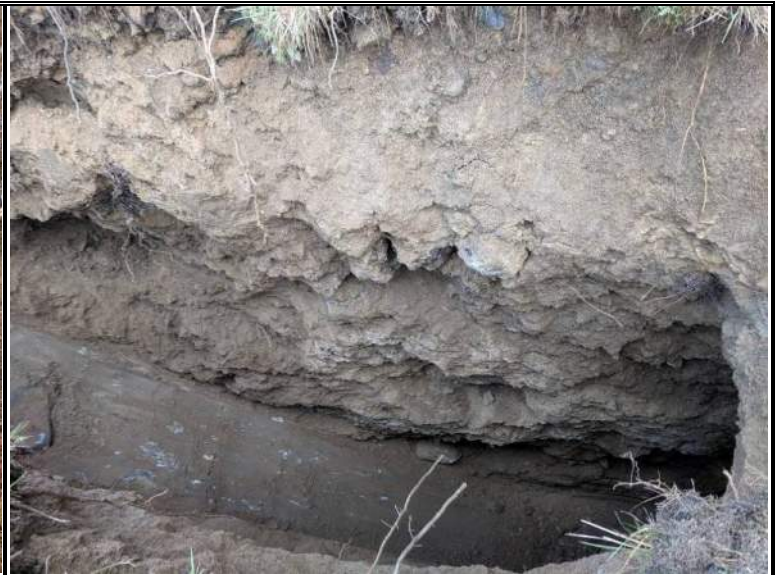
View of site conditions
