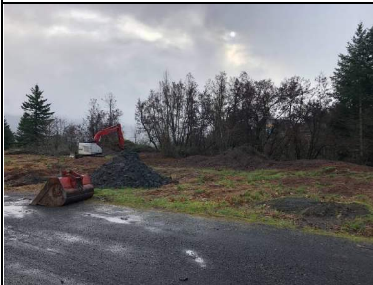
Excavation of test-pit TP-2, looking southwest
