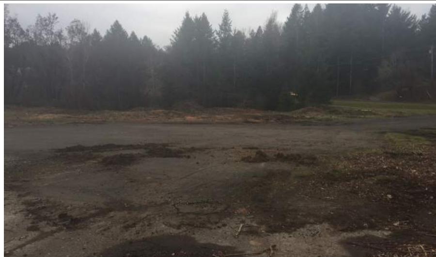
Photo 2. Existing concrete and gravel surfacing.
